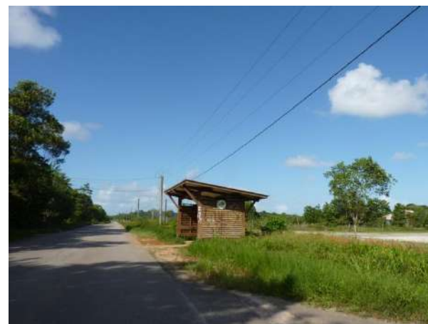
Figure 74: Abri bus Avenue Henri Kong
