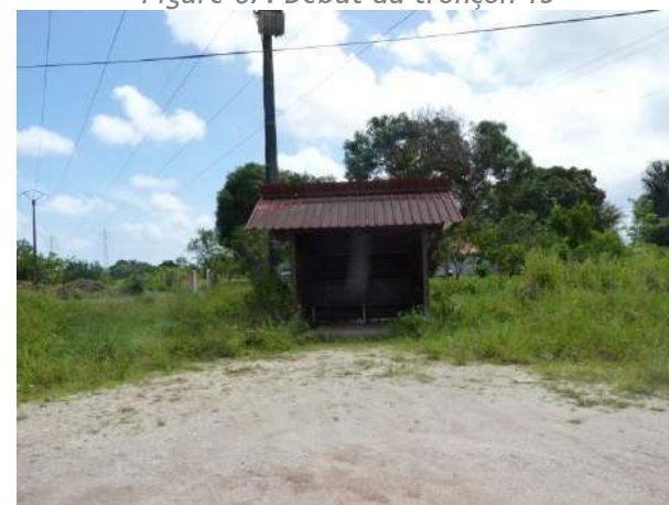
Figure 68: Abri bus proche de la RN1
